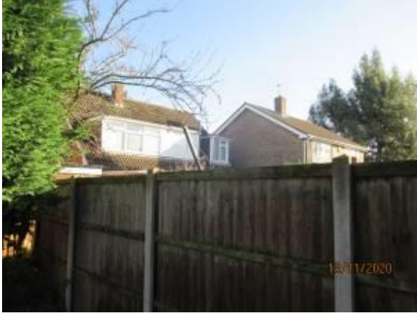
Rear elevation of 2 Rookwood Close
